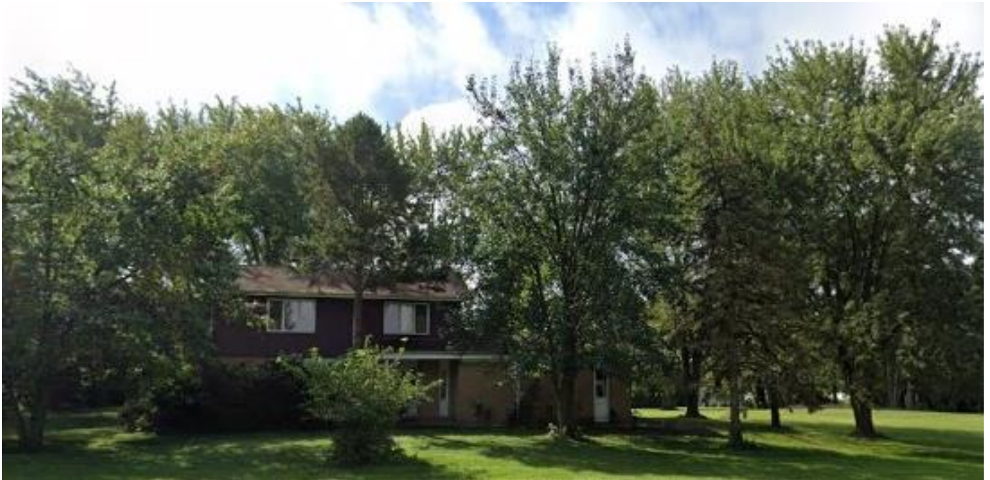
Home being renovated in Carpentersville
